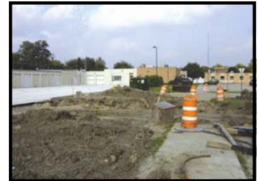
Ice Arena And General Services Building Parking Lot Construction.
